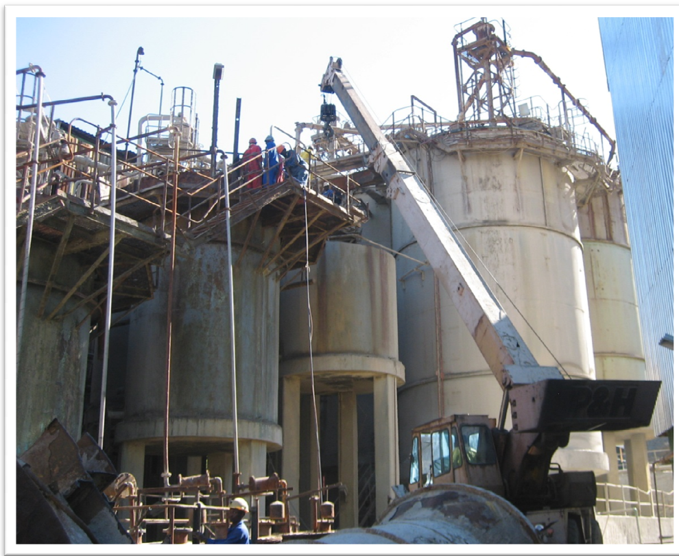
Plate 3: Plant personnel working at heights and others on the surface.
