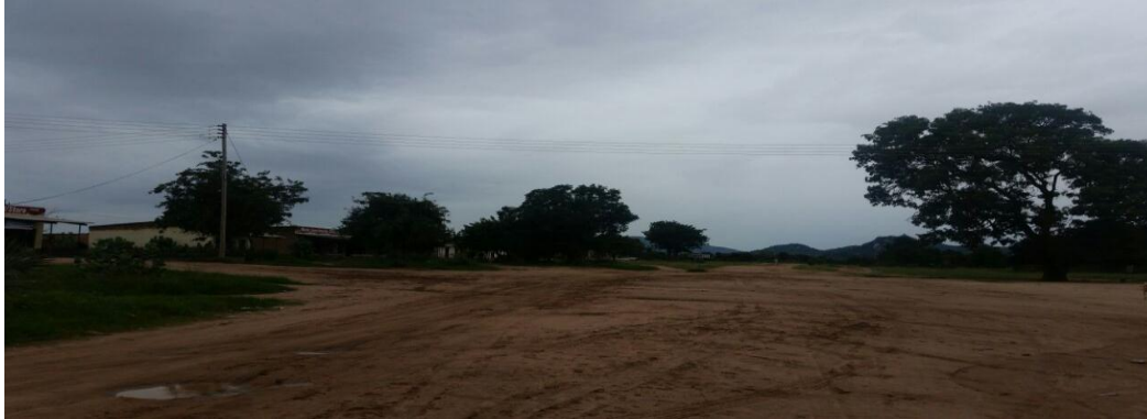
Fig 5: Graded road at Bambazonke Business Centre
