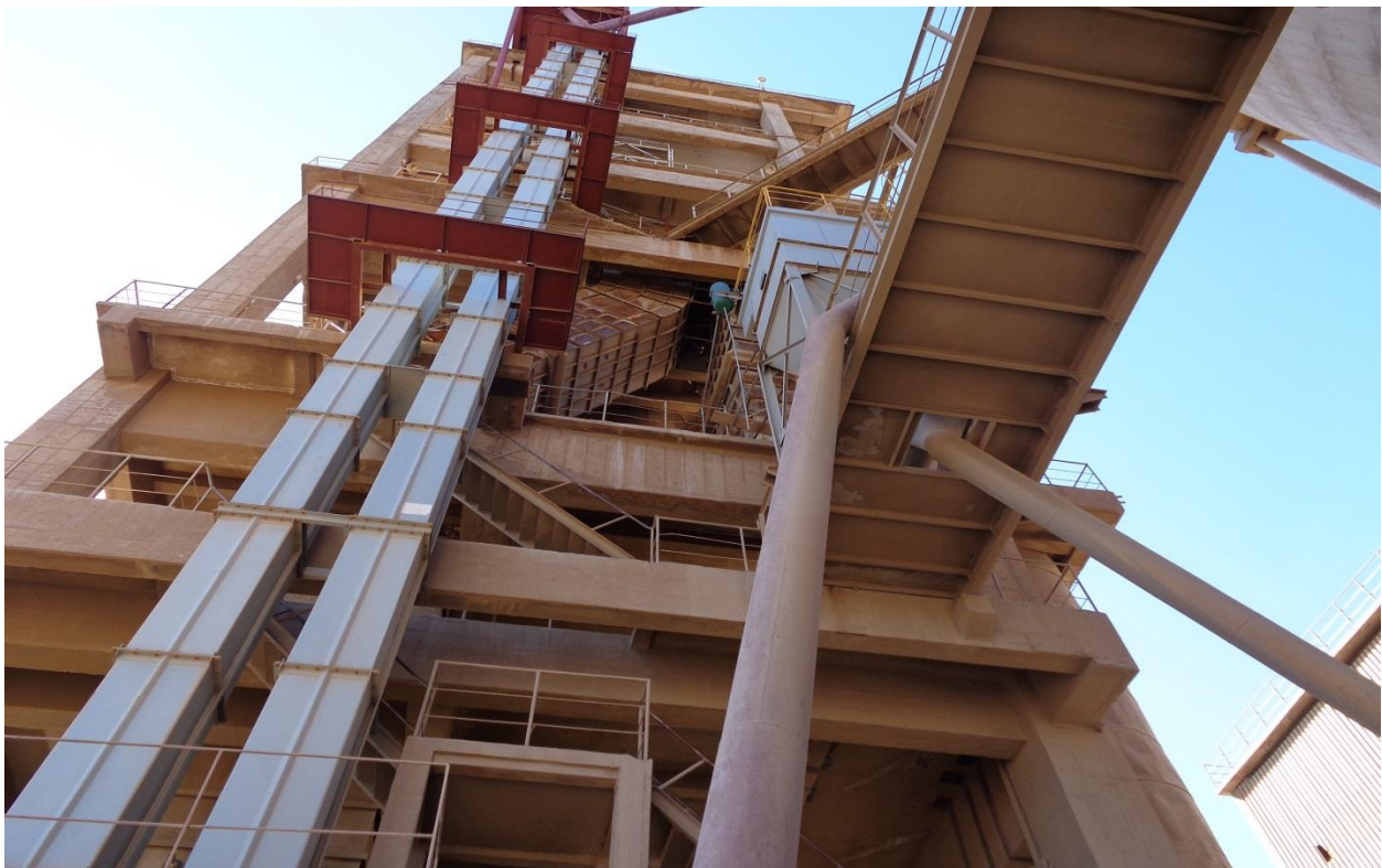
Plate 1: Sections of Grate Cooler Section (Source: SZCC S.H.E 2011 December report)
