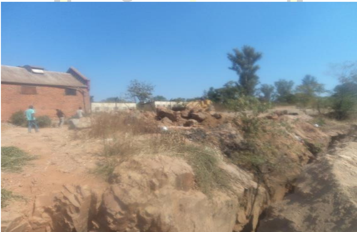
Unprotected shafts 10 meters away from the houses
