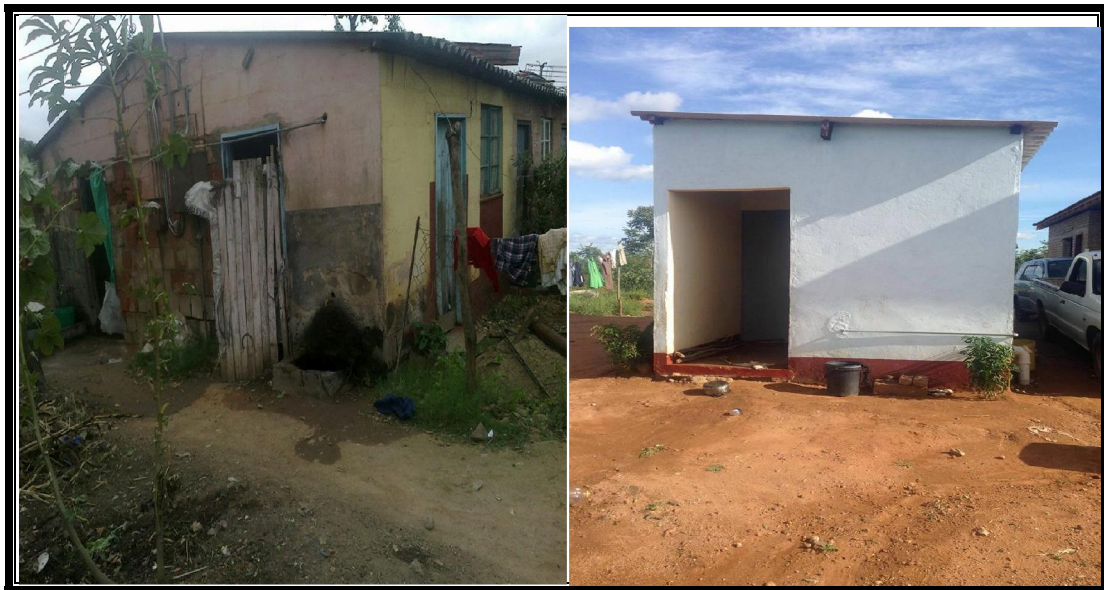
Plate 1: Mbizo 7 old housing units (left) Mbizo 22 newly constructed social houses (right)
