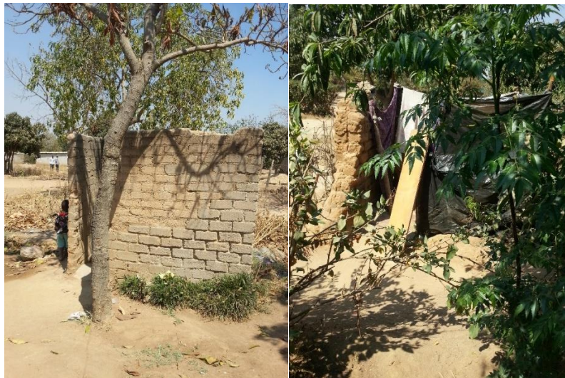
Plate 4. 2 Sub-standard toilets in Ward 7
