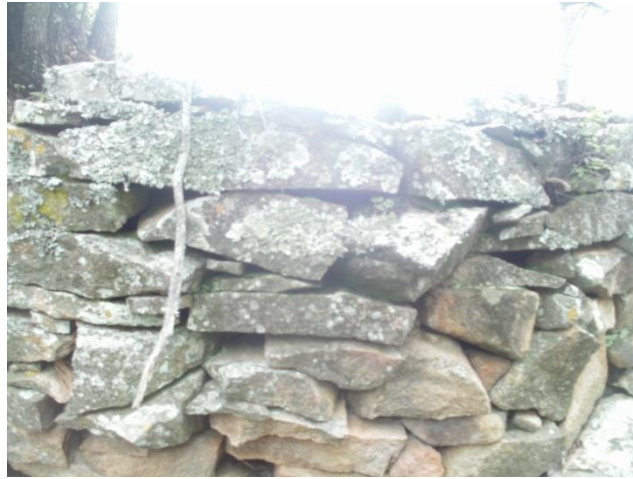
Photo 9 Western wall where the entrance is
