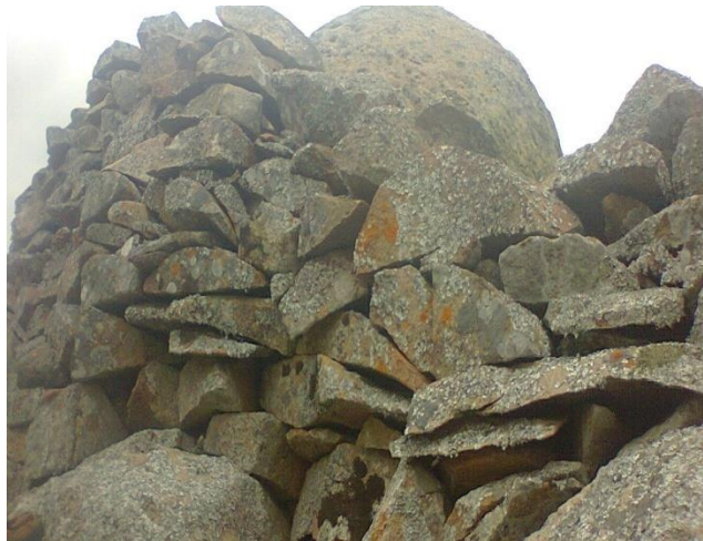
Photo 12 Part of the western walls.
