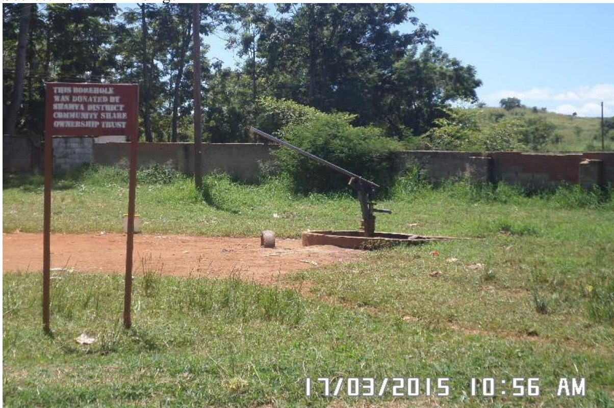
Borehole drilled in Wadzanai Township by the Shamva Community Share Ownership Trust
