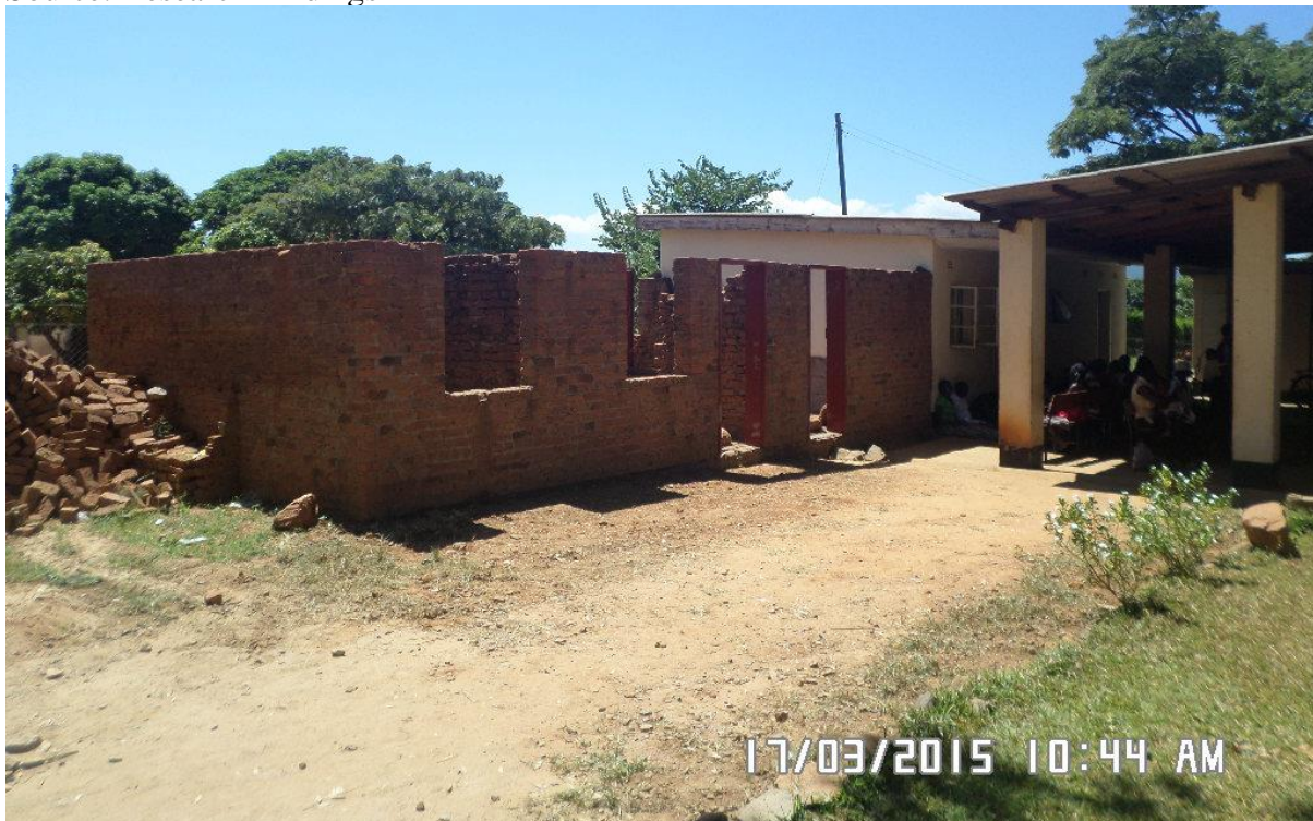
Mothers' waiting shelter being constructed at Wadzanai Clinic
