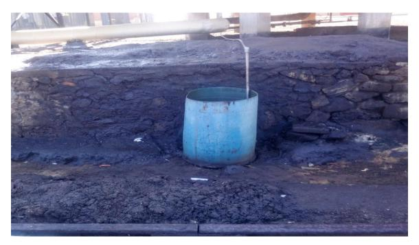
Plate 4.2: Oil pollution from the ammonia storage plant air compressor Source: Field data (2018).
