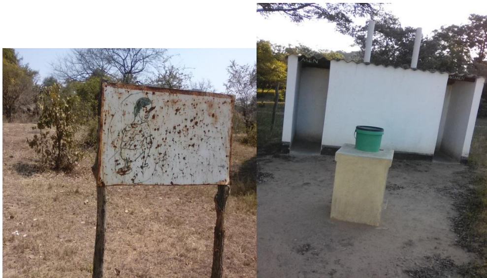
Fig 4. 7 Open defecation and Blair toilet
