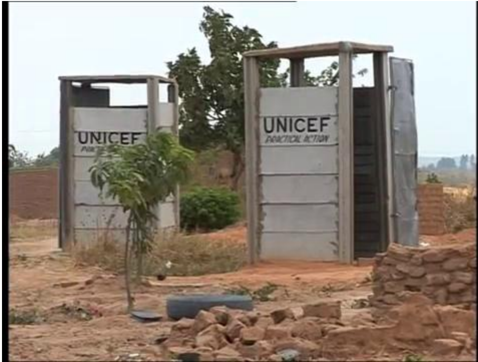
Plate 4.7: typical ecosan toilet facilities in Epworth
